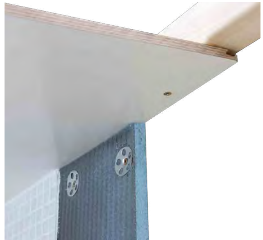
Wall finish with panels fixed to perimeter timber frame covered by tile backer/tiled surface
